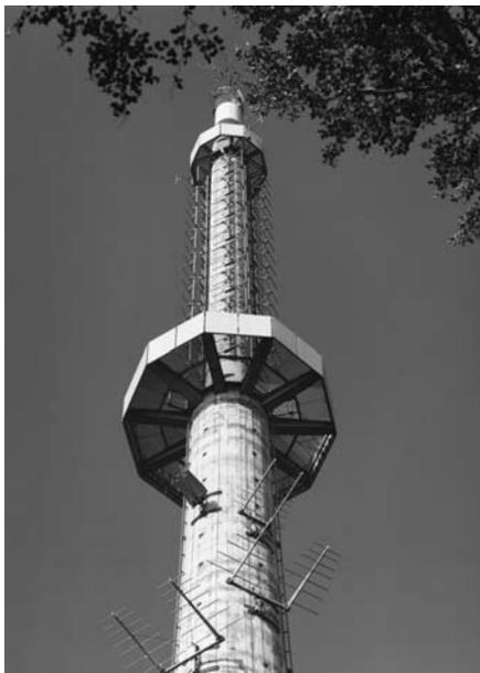
**FIGURE 29-19** Typical broadcast antenna installations on a concrete supporting structure. A UHF TV antenna is mounted on top of the tower. It is protected by a GRP radome that is provided with helical strakes to reduce its vulnerability to mechanical oscillation at certain wind speeds. Below this is a VHF FM radio antenna built from dipole panels, and below this is a variety of LPDAs. (Courtesy of Kathrein-Werke KG)
